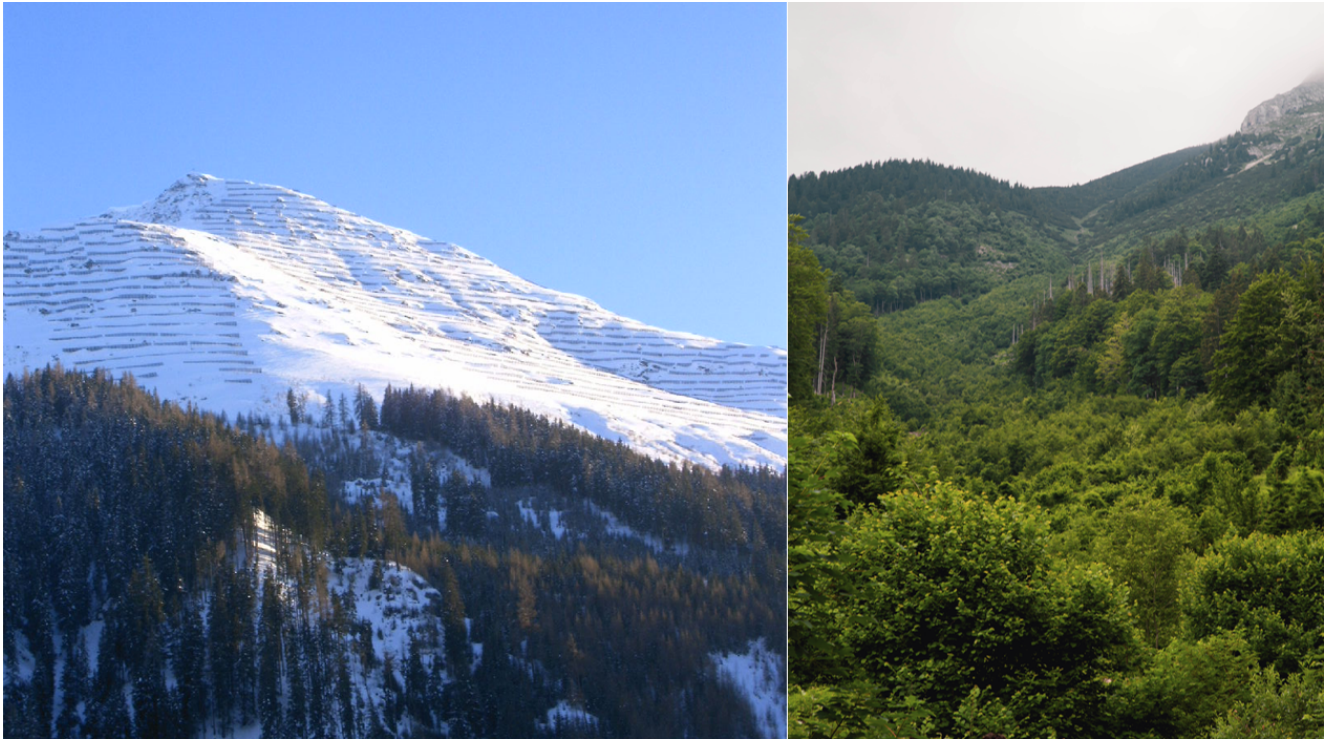
Figure 67-4: Left: Artificial avalanche protection measures on the mountain slopes above a protective forest. Right: Avalanche path in an Austrian mountain forest.
